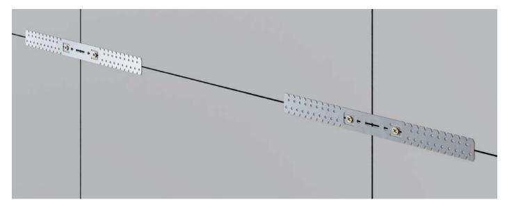
3. Align one edge of the profile with the marked line and drill holes for expansion plugs using a perforator. Attach the profile. The profile should be secured at a distance from the wall equal to the thickness of the mineral wool, recommended at 50 mm for optimal sound insulation and absorption.
