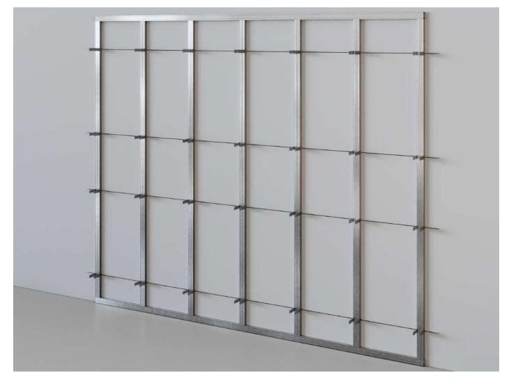
6. The hangers are fixed at a distance of 600 mm from each other. It is customary to reinforce the profile when assembling the wall frame with a spacing of 600 mm and the installation of transverse stiffening ribs – this is a standard scheme for positioning load-bearing posts.
